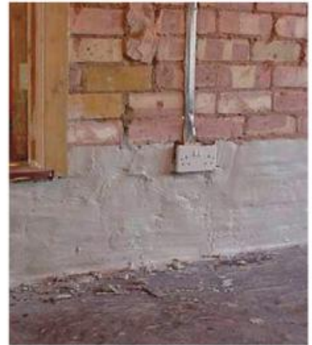
Slurry Coat Waterproofing for wall areas below dpc level e.g. steps in floor level
